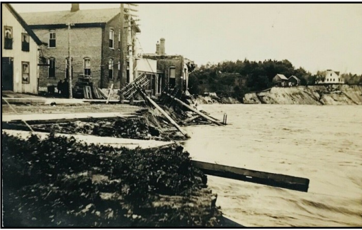
In rapid succession, brick, stone and frame buildings were undermined by the water and slowly crept into the river.
