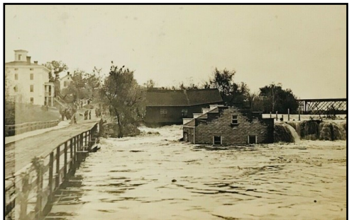
Flood damage at Black River Falls, Wisconsin October 1911.
