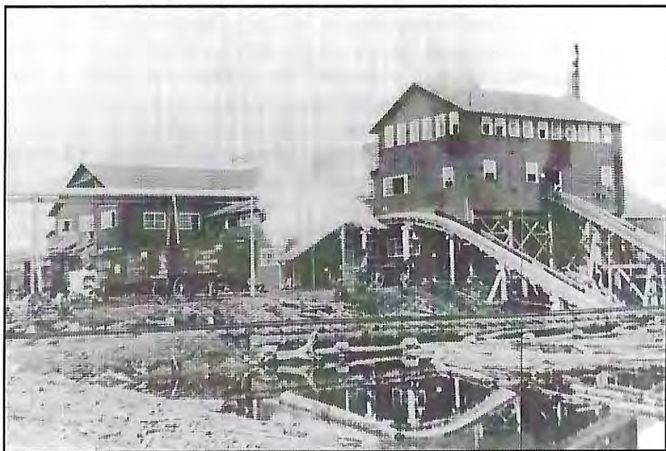
Front view of the Menominee Bay Shore Lumber Company.
