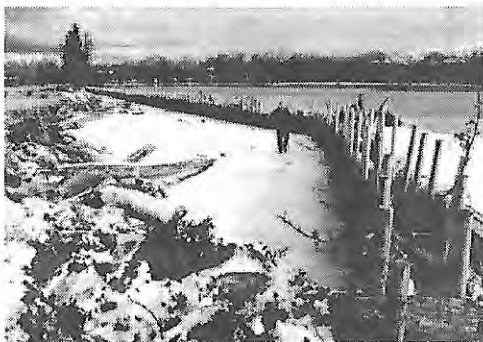
Mark Lorang walks along the edge of an erosion wall at a waterfowl production area on the Flathead River near Flathead Lake. The 600-foot long wall is made from more than 3,000 recycled Christmas trees. More trees are being gathered this year.
