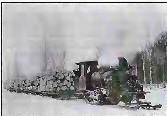
Steam log hauler made by Phoenix Manufacturing Company of Eau Claire, pulling loaded skids through snow. Rice Lake lumber camp, overland spur, ca. 1914. Wisconsin Historical Society.
