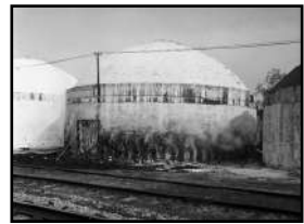
Smoking Charcoal Kiln: A typical railroad charcoal kiln. Note the door at the bottom and the smoke coming from the row of vents along the bottom. (Ohio Agricultural Research and Development Center).
